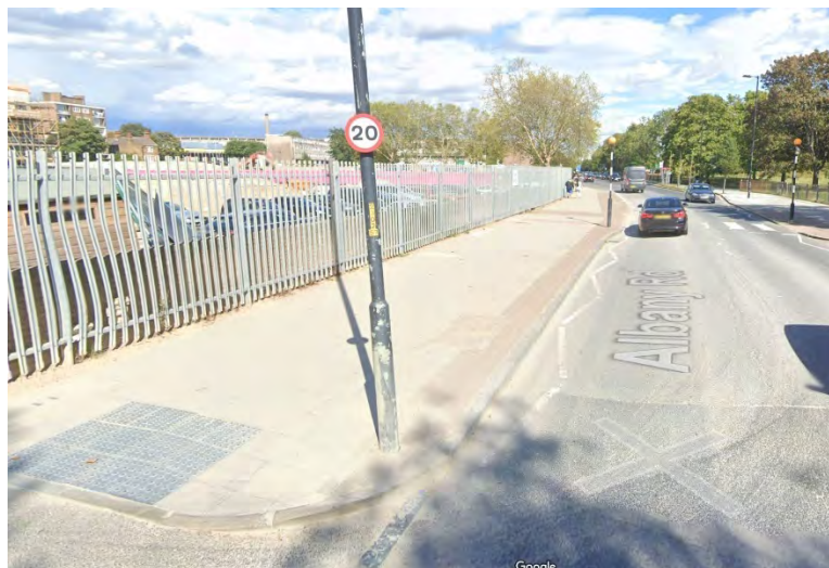
Photo 1: Albany Road Adjacent to Footway FDS Southern Boundary
